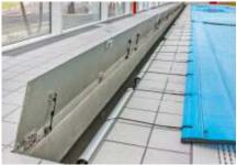
Blanket roller shall be of anodized aluminium and clear-span for the width of each pool cover with allowance for cover "run-out" mounted by a 12mm Aluminium endplate and suitable bearing.
